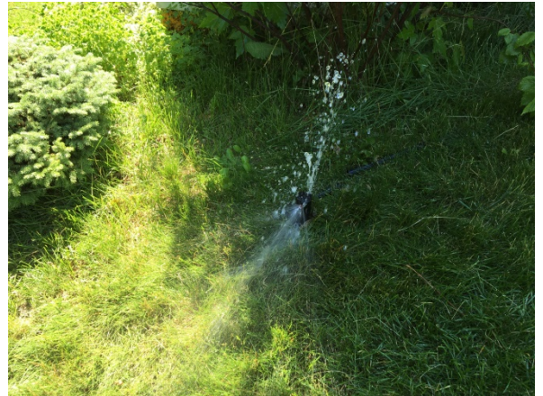
REPLACE BROKEN AND LEAKY SPRINKLERS
